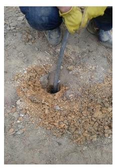
11-09-2016-002: Bentonite grout was applied to the wells after removing the well casing and screen and was allowed to sit overnight to account for settlement.
