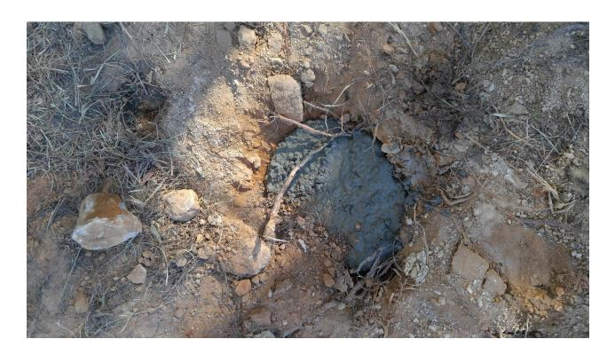
11-10-2016-001: A concrete cap seal was poured on top of the bentonite grout after allowing the grout to settle.
