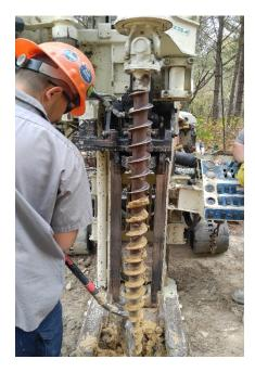
11-09-2016-001: GeoLab used the geoprobe to over drill wells to remove the casings that broke or were not able to be completely removed.
