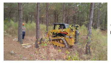
11-08-2016-001: A skid steer was used by the GeoLab to break up the concrete pads and pull the PVC well casing.
